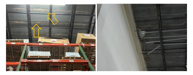
Photo shows significant corrosion of roof decking
